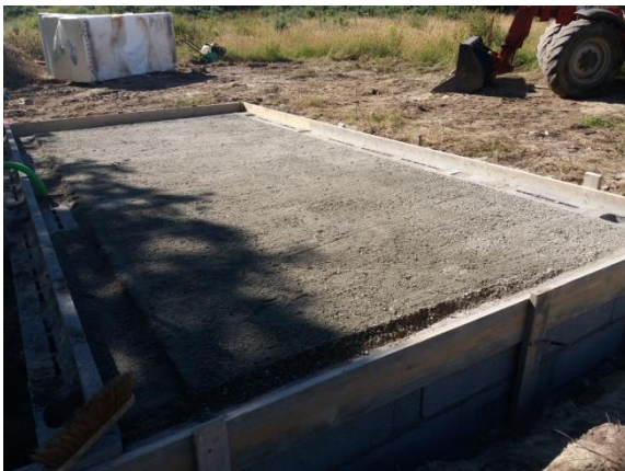
Figure 44 : Remblayage dalle
